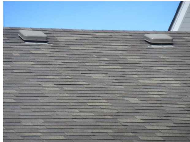
Laminate shingles and box vents at roof peak
