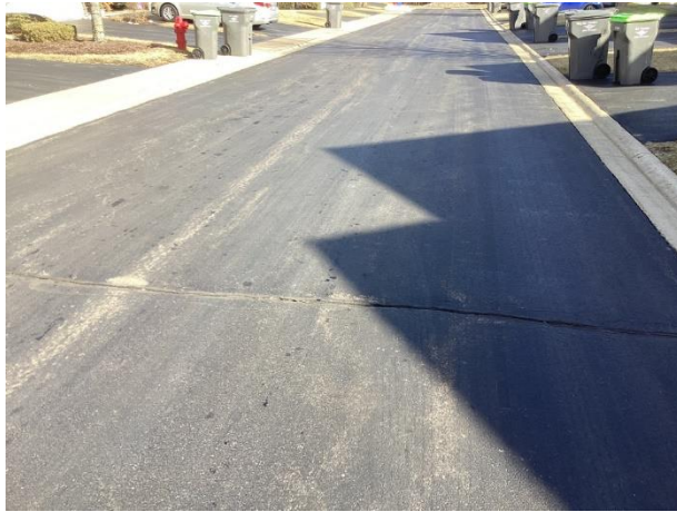
Access drive overview with repaired transverse cracks
