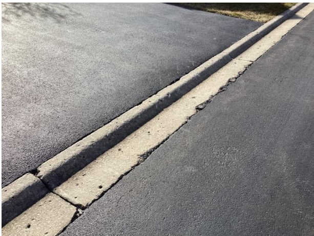
Concrete spall at mountable curb and gutter section
