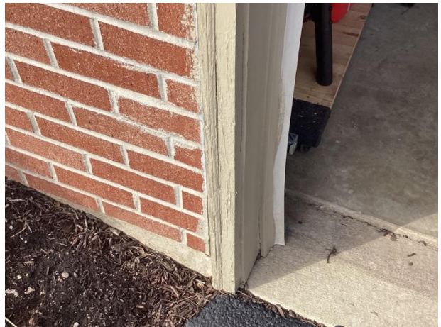
Deterioration at garage door trim
