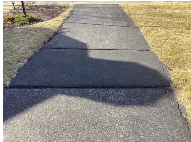
Repaired transverse cracks
