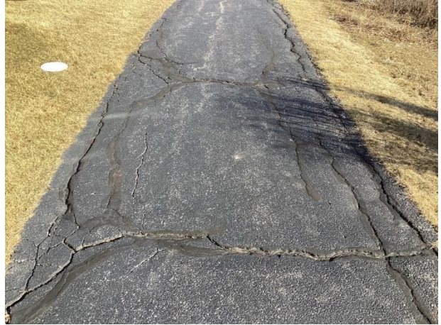
Cracks and settlement
