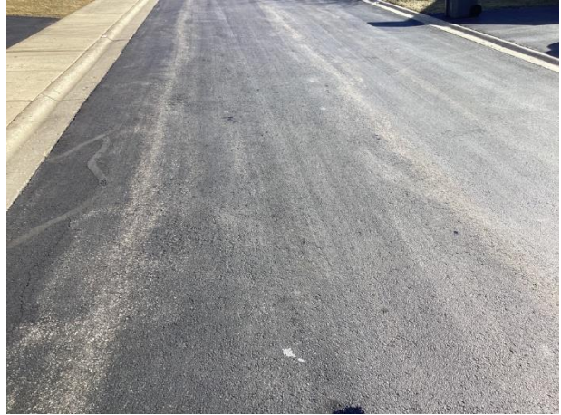
Repaired cracks at pavement edge
