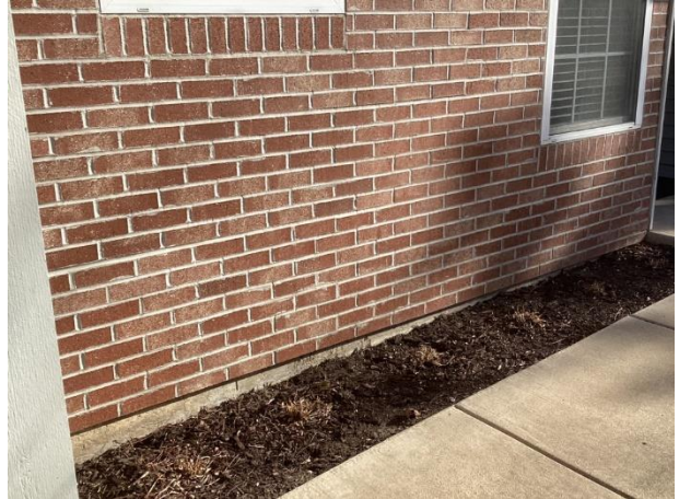
Section of thin brick veneer in good condition
