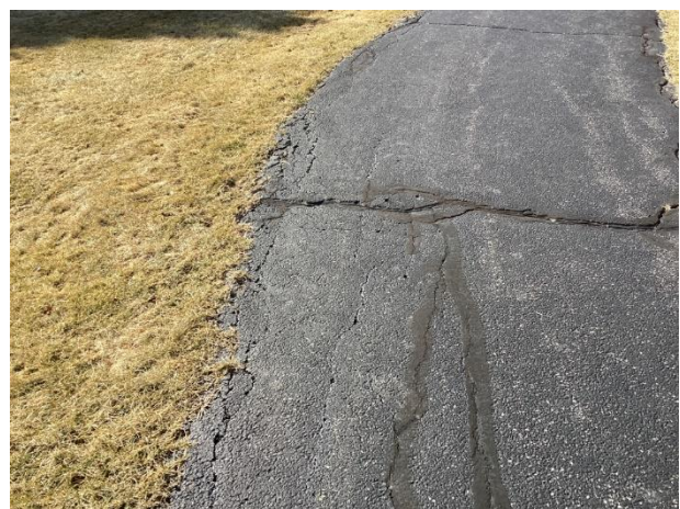
Significant deterioration at south section walking path near the pond
