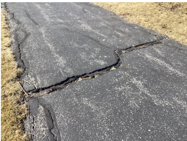
Wide asphalt crack and previous repairs
