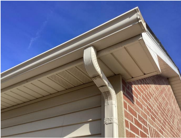
Aluminum gutter and downspout
