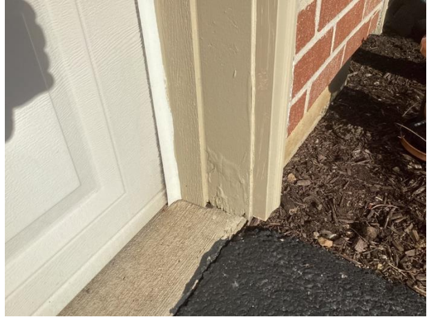
Deterioration at garage door trim
