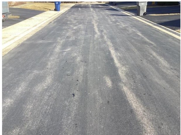
Seal coat fade
