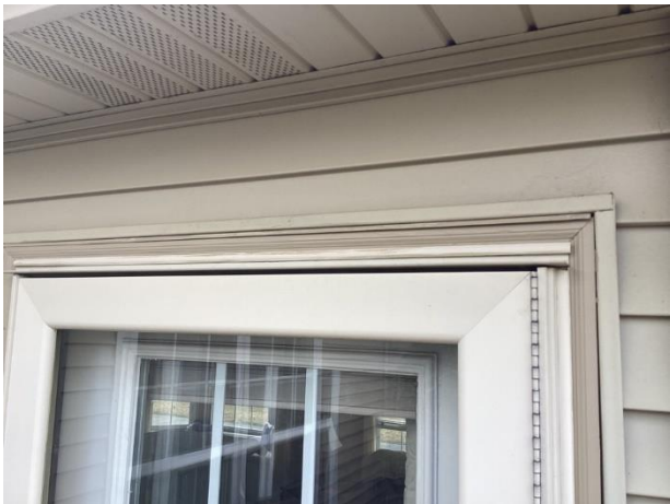
Wood trim present at rear elevation doors
