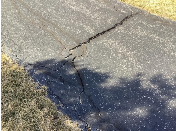
Wide asphalt cracks
