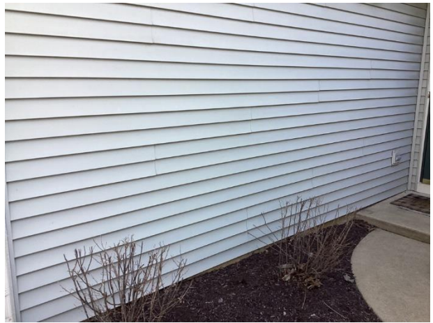
Typical condition of the siding with color fade but no deflection or damage
