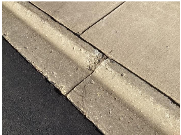
Deterioration at control joint
