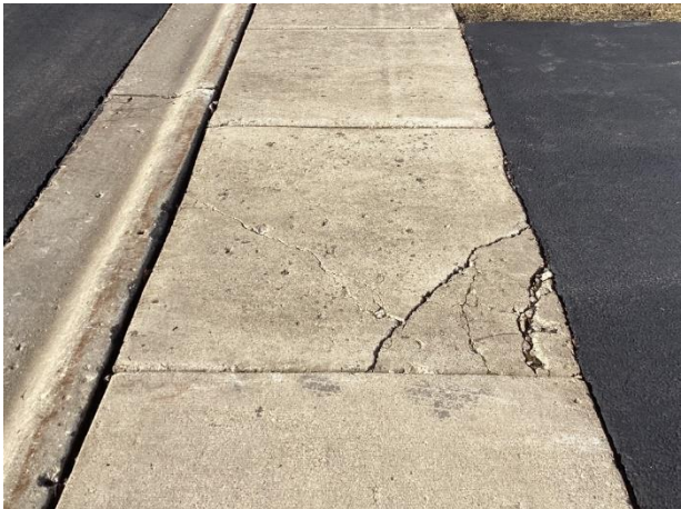
Isolated sidewalk cracks adjacent to driveway
