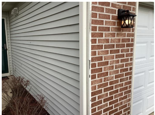
Wood trim deterioration
