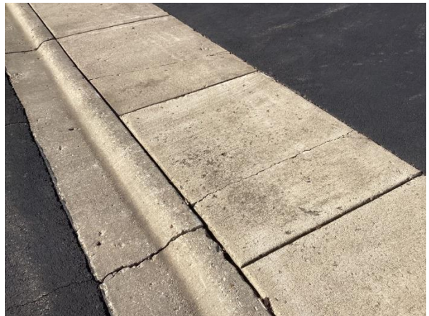
Concrete flatwork cracks
