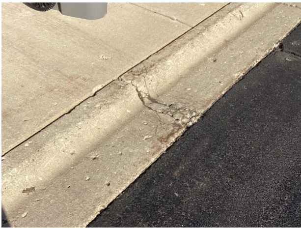
Curb and gutter cracks and deterioration
