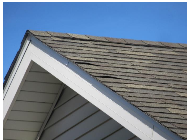
Shingle lift at gable roof edge
