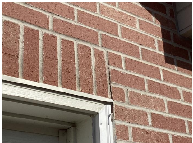
Significant mortar cracks
