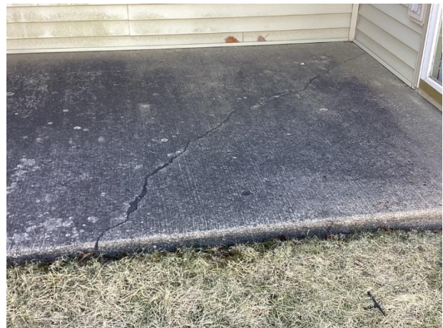
Isolated patio crack
