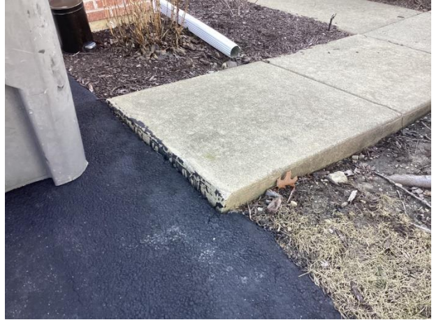
Level discrepancy between driveway and sidewalk
