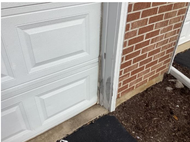
Significant finish deterioration
