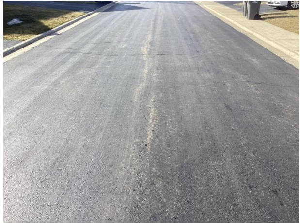
Crowned asphalt pavement at access drive with seal coat and previous repairs
