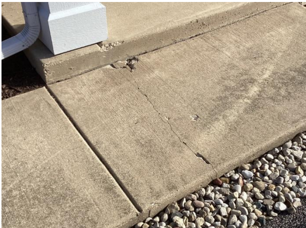
Cracks and spall
