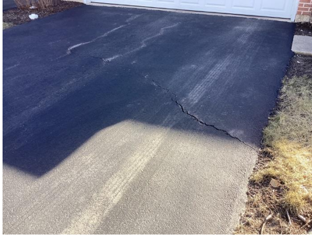
Significant unrepaired crack
