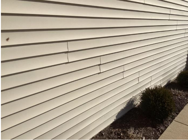
Vinyl siding with a clapboard profile
