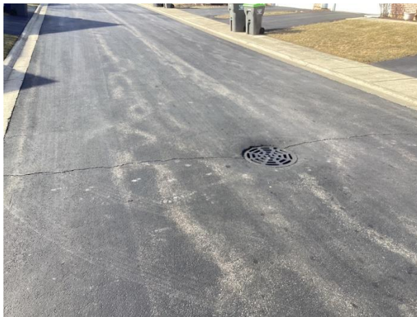
Transverse cracks
