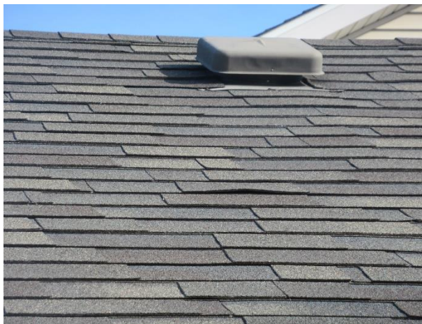
Isolated shingle lift
