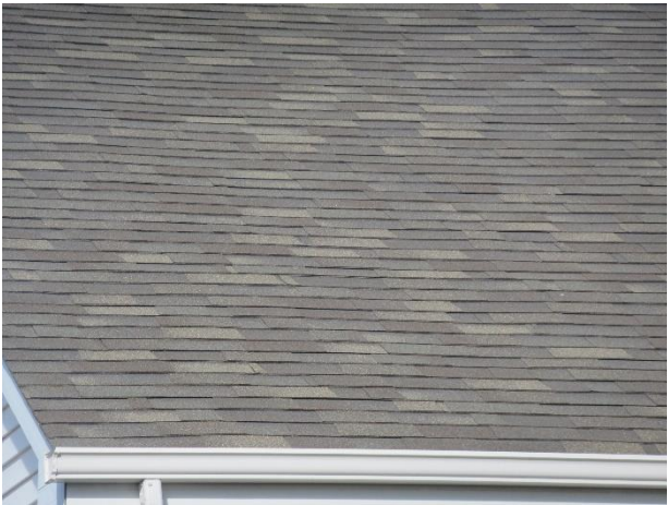
Laminate asphalt shingle roof
