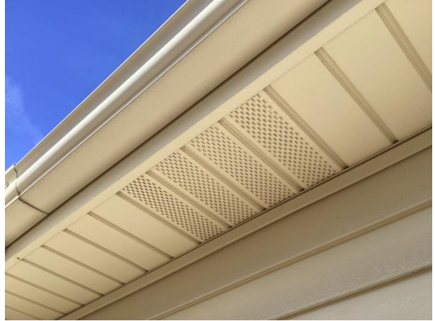
Perforated aluminum soffit and fascia
