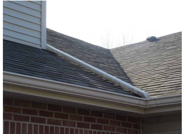
Downspout discharge from upper roof section directly into lower roof section gutter
