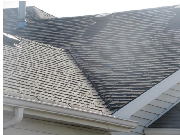
Isolated instance of shingle bulge and lift adjacent to valley
