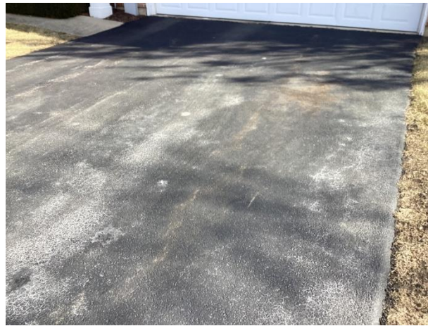
Cracks, settlement and vehicle fluid stains
